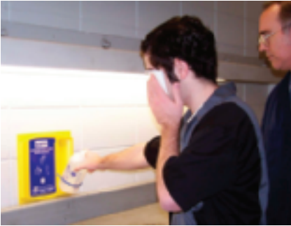
P1-1 Remove the eyewash bottle from the wall holder. The injured person may require assistance.
